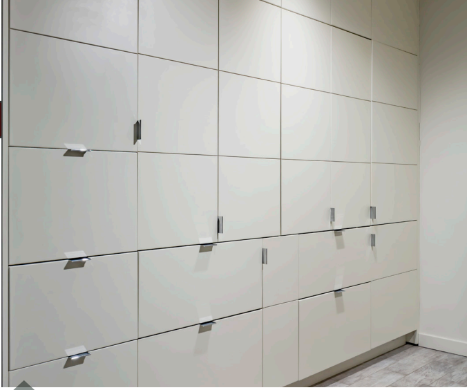
The concealing door and drawer panels can be painted or stained wood, or plastic laminate.
